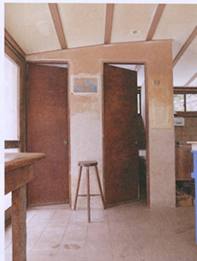
Rear section of the Conoid Studio, with its distinctive conoidal shell roof in reinforced concrete, designed by Nakashima in 1957 (1)
